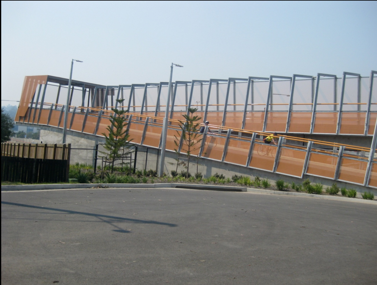
Overpass for cyclists and walkers – Pacific Highway, Brisbane, Australia
