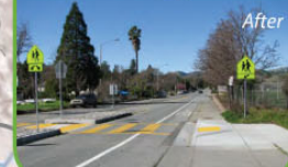
Novato: "Complete Street" improvements on Olive Way serving Olive Elementary
