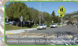
Novato: Curb extensions, signage, and high visibility crosswalks to San Ramon Elementary
