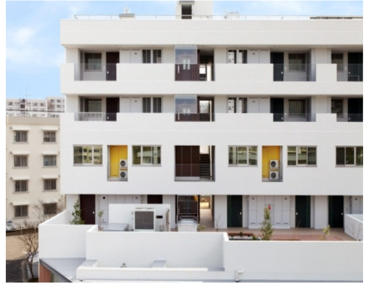
the north view
